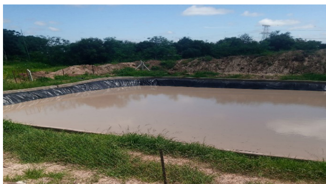
Rain water harvesting structure supported by ASDSP II
