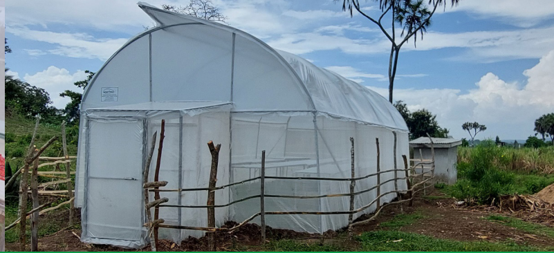
An outside view of the 2 MT per week solar drier established at Matokeo Women Group in Kubo South, Kwale County
